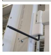
3. Pressure adjustment: Remove the cap from the top of the hinge. Use an 8mm hex key to turn the plastic insert to increase/decrease the pressure on the door seals.
