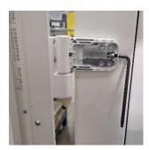
2. Vertical adjustment: Use a 5mm hex key to turn the screw from the bottom of the hinge.
